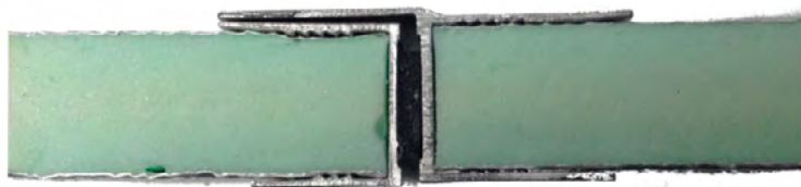
Connection system with aluminium profiles.
