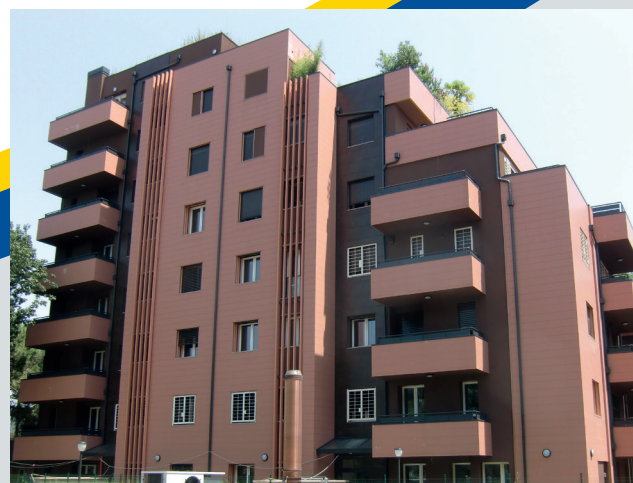
Mixed solution with external thermal insulation and ventilated façade (STIFERITE Class SK and Fire B)
