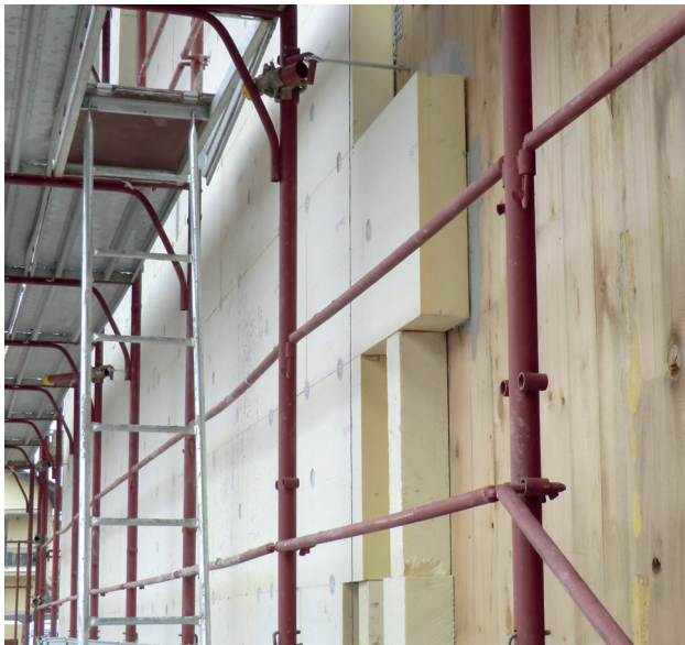
External thermal insulation on wooden structure
