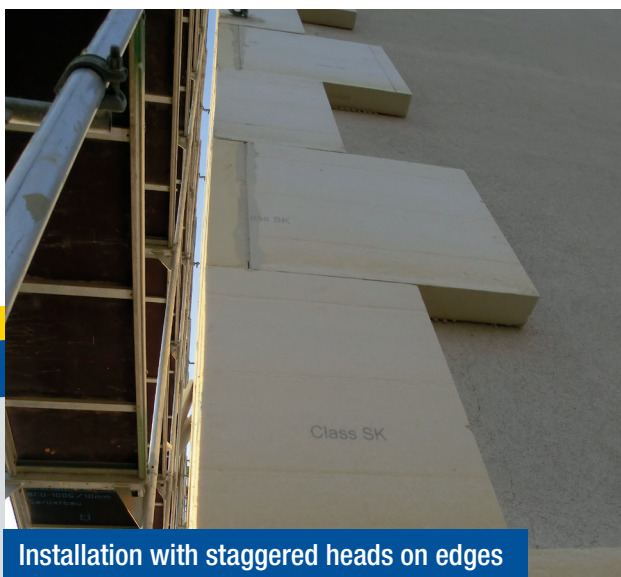
Mixed solution with external thermal insulation and ventilated façade (STIFERITE Class SK and Fire B)
