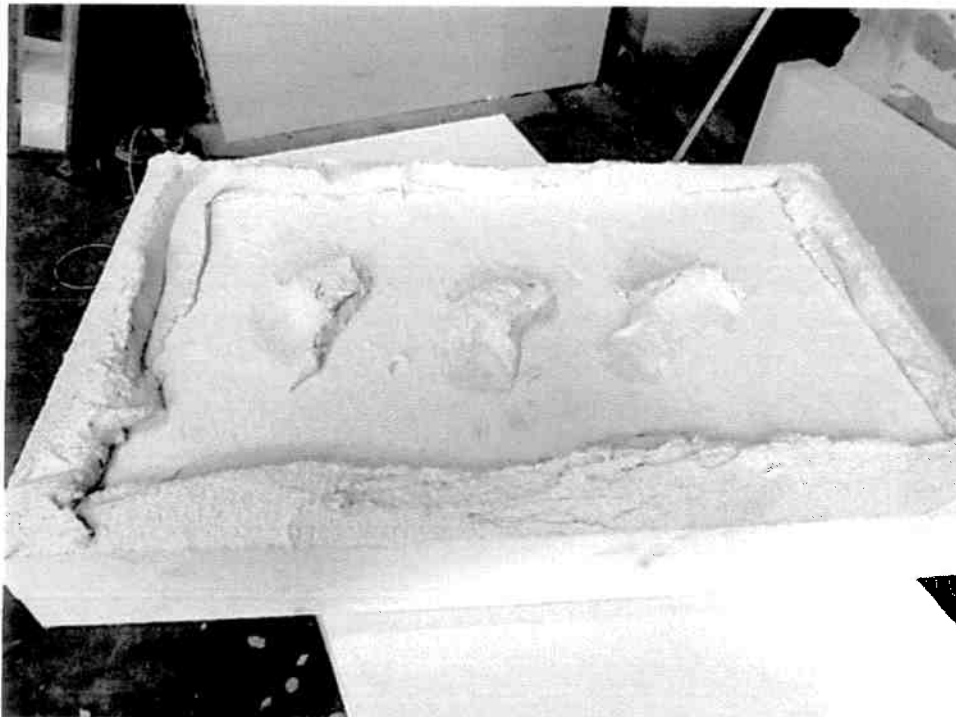
Picture 2 (P1010494): Application of adhesive to insulation board
