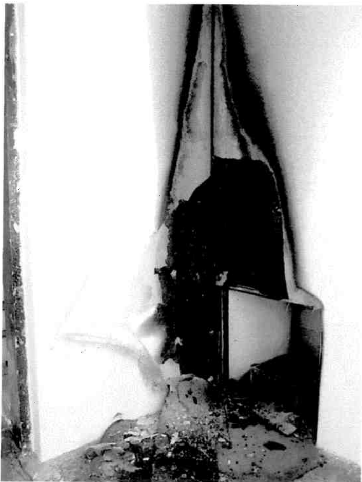
Picture 19 (P1060141): Test specimen after testing, with rendering removed
