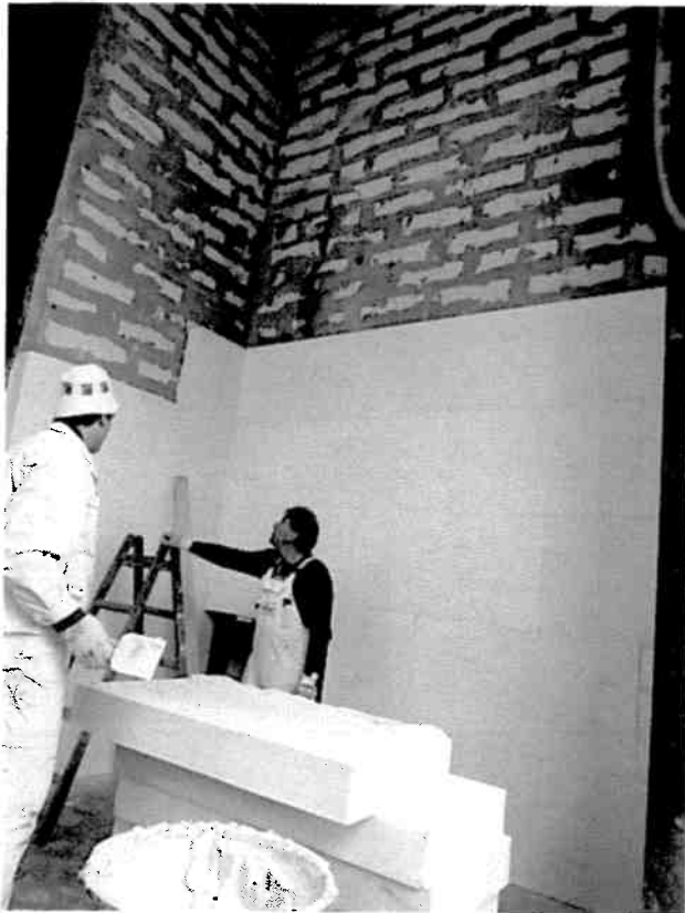
Picture 4 (P1010529): Textile glass mesh being applied
