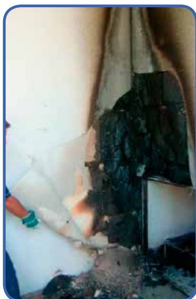
Removal of the plaster layer in order to verify the state of the insulation. STIFERITE's Class SK is charred only in the zone exposed to the flame.
