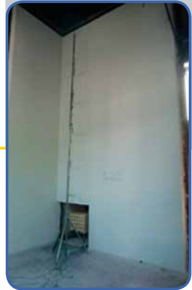
The test on a 6 meter wall in conformation angle.
