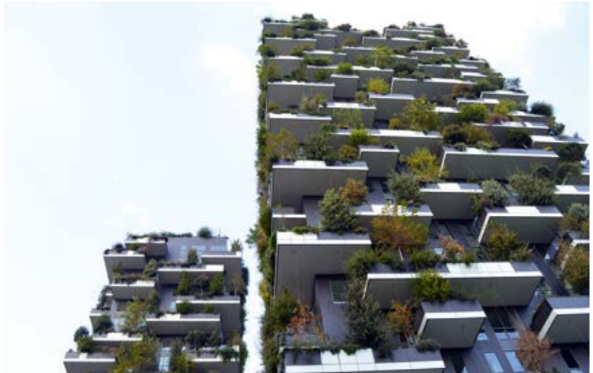
Bosco Verticale, Milano LEED® Gold STIFERITE GT, Class B
